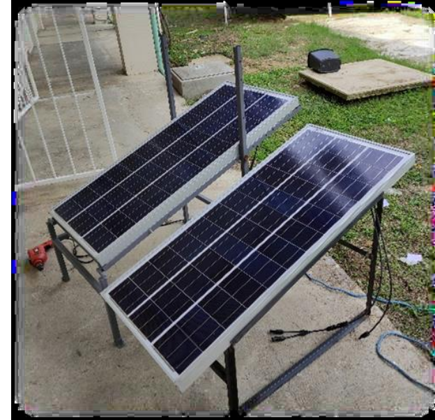
Installation: For panel-frame mounting, stainless steel screws are required; four holes are made in the solar panel frame.
